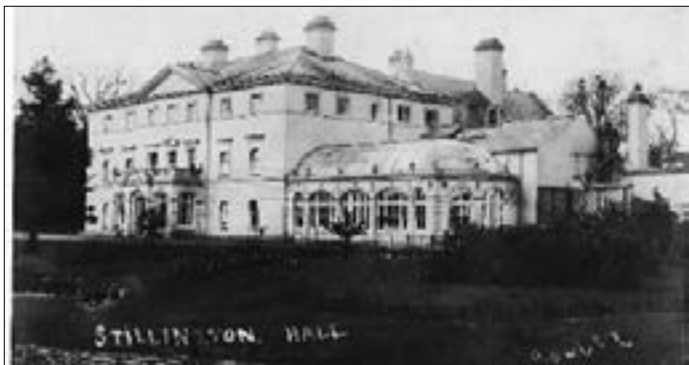
Figure 1. Stillington Hall, demolished in the 1960s was the scene of William Hemsall's notorious burglary in 1847.
