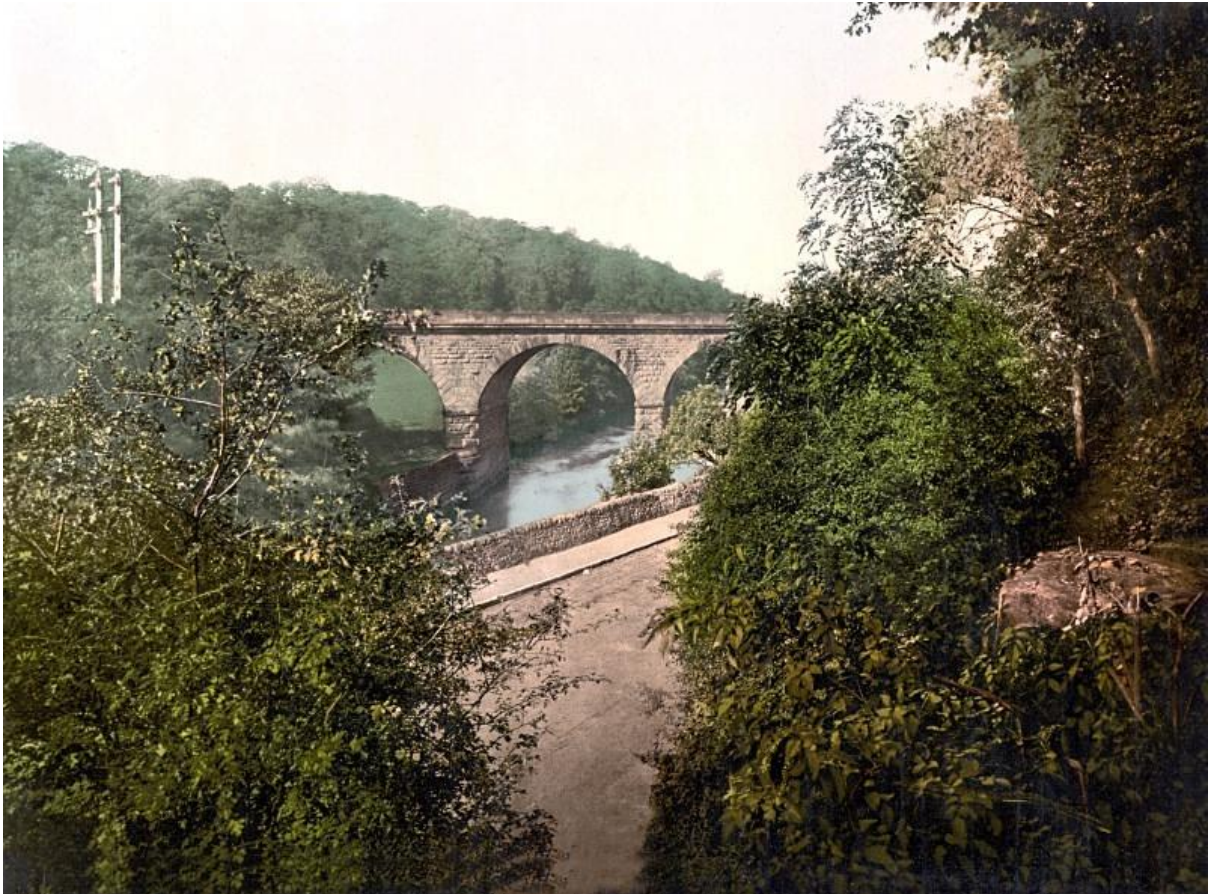
The railway bridge at Ambergate, Derbyshire.
